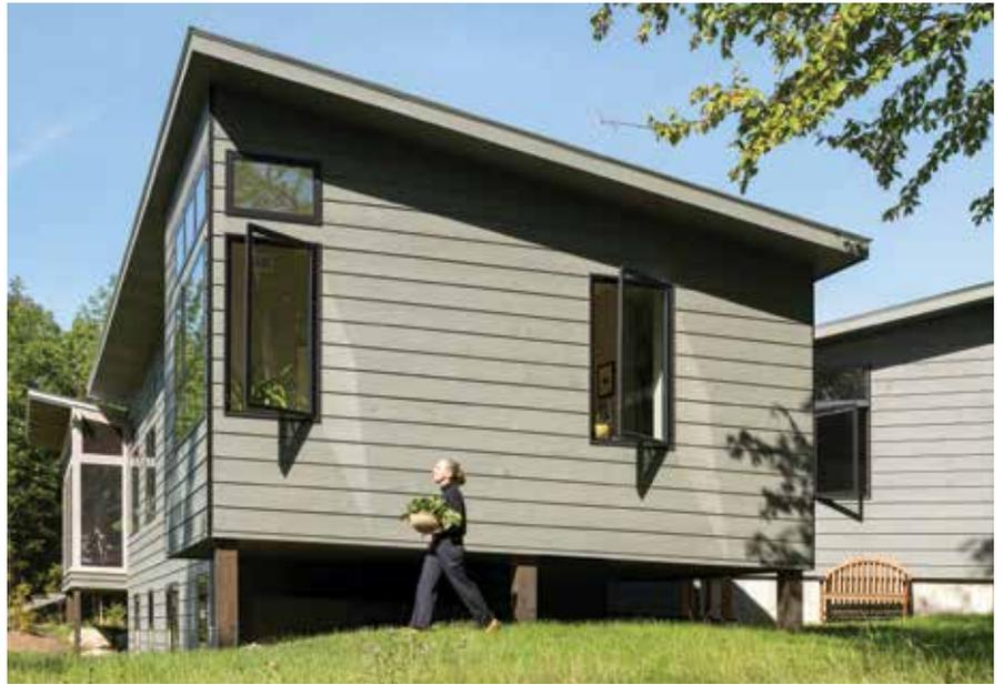
*TO TREAD AS LIGHTLY AS POSSIBLE ON THE LAND, THE SCREENED PORCH AND BEDROOM ARE BOTH BUILT ON POSTS OVER LEDGE IN THE GROUND.*
